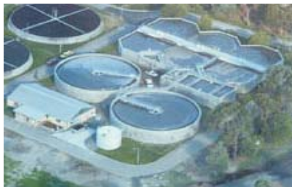
Figure 10.7 An aerial view of a sewage plant
